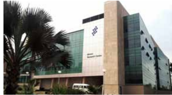
Biocon R&D Building Water-cooled Screw Chiller India
