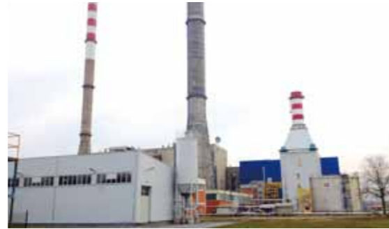
Sisak Thermolectric plant Air-cooled Screw Chiller; GMV Croatia
