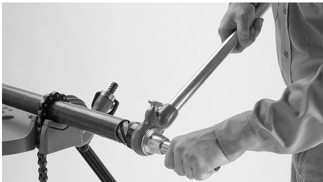
Figure 2 – Reaming End of Pipe
